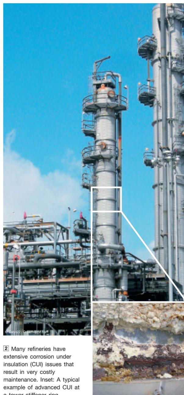
[2] Many refineries have extensive corrosion under insulation (CUI) issues that result in very costly maintenance. Inset: A typical example of advanced CUI at a tower stiffener ring.
