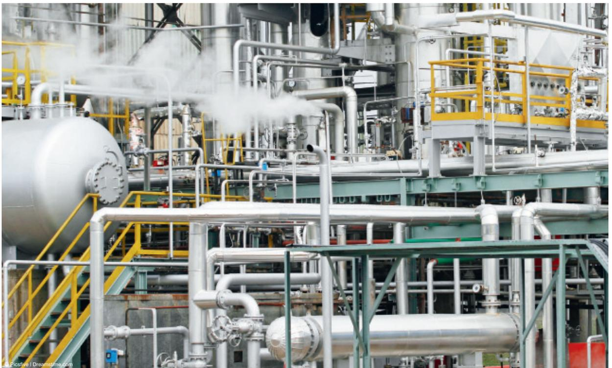
[1] Section of a refinery—the piping can be exposed to aggressive fluids under the insulation.
