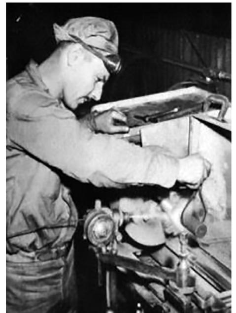
Figure 2: Combustion wire spraying with a Metco gun back in the mid 20<sup>th</sup> century.
