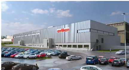
Caption: Exterior view of the new Oerlikon Barmag production building on Leverkusenerstrasse in Remscheid Lennep.
