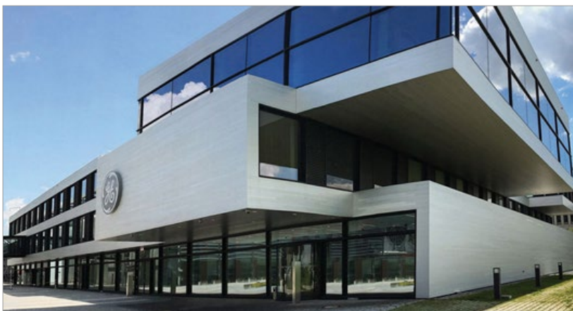
GE Additive's Customer Experience Center is co-located with GE's European Technology Center in Munich, Germany
