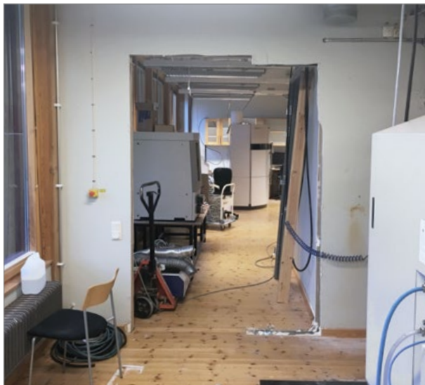
Fig. 4 A doorway has been widened to move an AM system into place (Courtesy Olaf Diegel)
