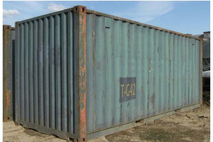
Corrosion caused by weather and exposure
